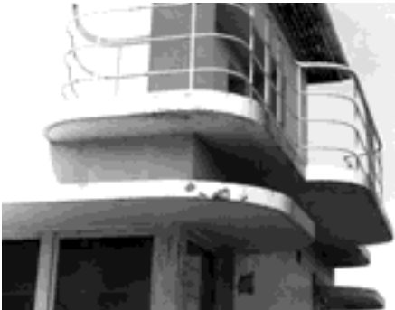
Former Pilot Station Outer Harbor
