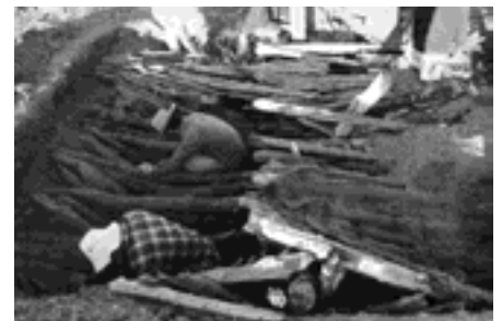
Work on miner's dugout, Appealinna Mine Flinders Ranges
