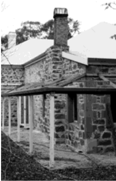
Re-roofing Wilpena Homestead
