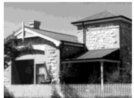
Former Semaphore Fire Station
